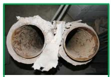
Contractors installing the new HVAC system throughout the Capitol are replacing worn, corroded pipes such as these.
